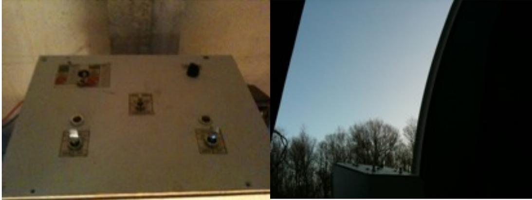
*Figure 28 (Left) and 29 (Right): Dome Doors control panel and successful opening. Note the positions of the doors with respect to the Sun (Spring Equinox); in this position the dome has its solar panel pointed to the Sun during the afternoon hours, allowing the battery to complete its charging cycle by dusk.*
